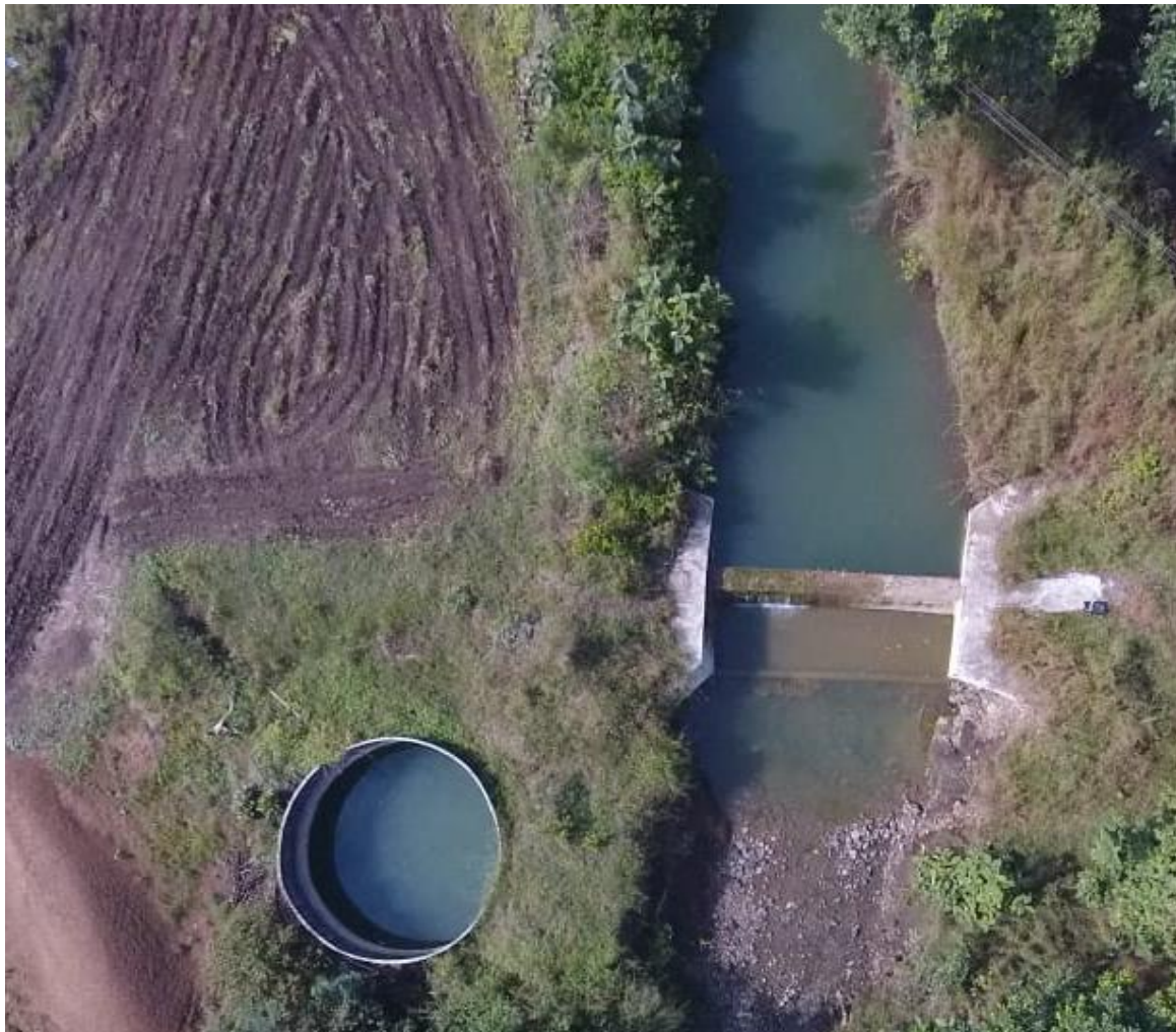
Check Dam and dug well at Skikarpur, Sehore District
