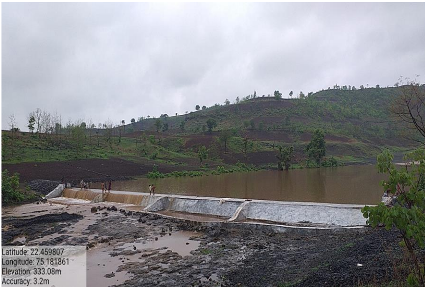
Check Dam at Khirkiya Kalan, Block Tirla, Dist. Dhar.
