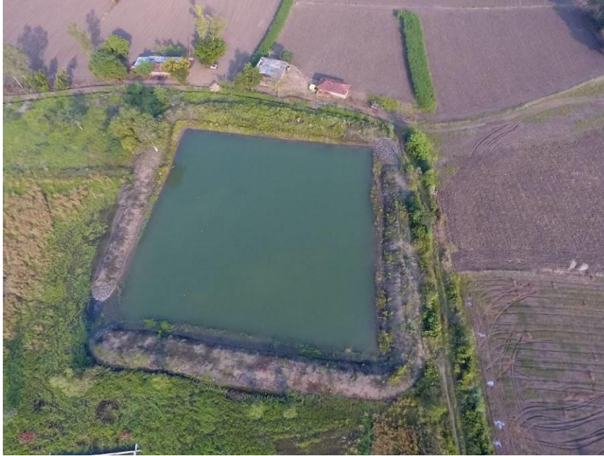
Farm Pond for irrigation at village Dhabla, Dist. Sehore. Water Storage Capacity 9039Cum. Command Area 18.08 ha.
