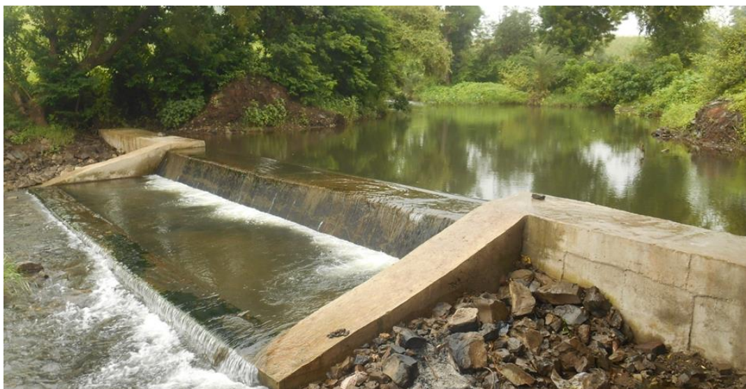
Check Dam at Badlipura kalan, Tirla Block, Dhar District
