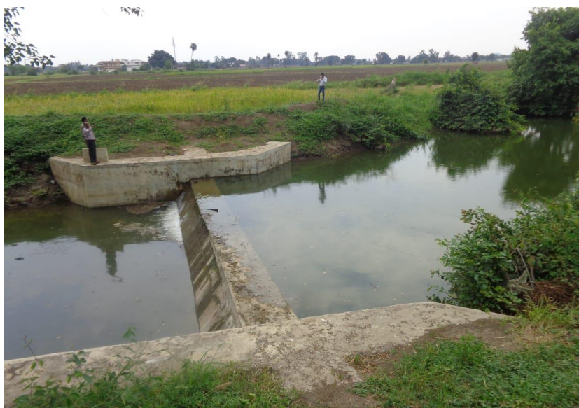
Check Dam across Kolans River at Barwakhedi
