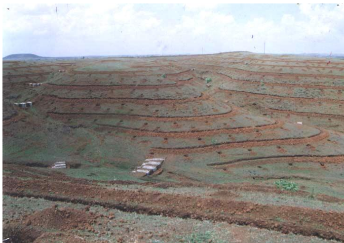
Continuous contour Trenches (CCT) and gully plus under RGM watershed project in Khardubadi village in Jhabua block of Jhabua district.
