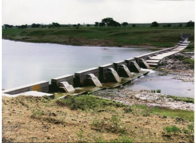
Construction of stop dam at Govindpura village of Sardarpur block (Dhar dist.) under RGM (DPAP VI th batch)
