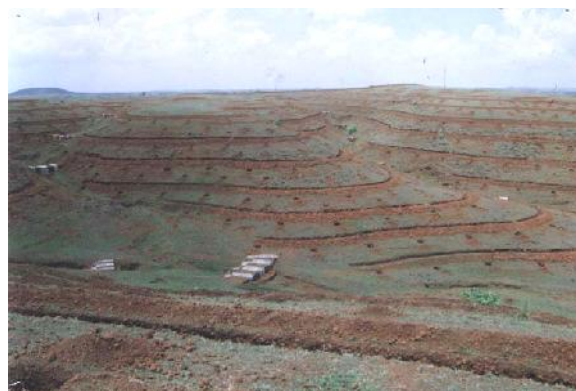
Continuous contour Trenches (CCT) and gully plus under RGM watershed project in Khardubadi village in Jhabua block of Jhabua district.
