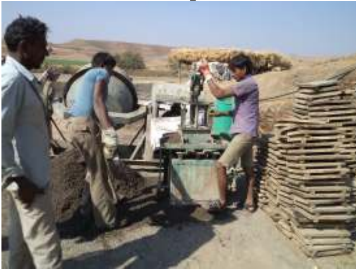
Concrete cement blocks, Vandana watershed Self Help Group, Vaglawat, Jhabua
