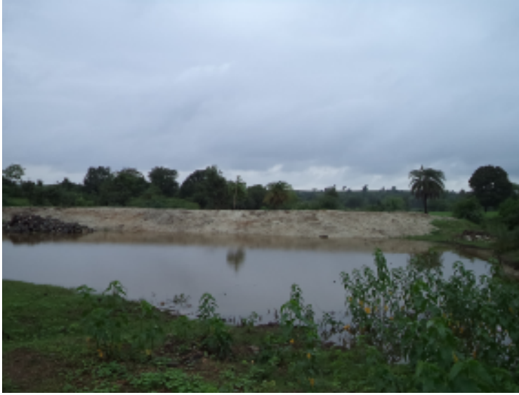
Earthen Dam, Cost - Rs. 1.78 lakhs Irrigated area – 9.63 ha. Village – Tichkiya.
