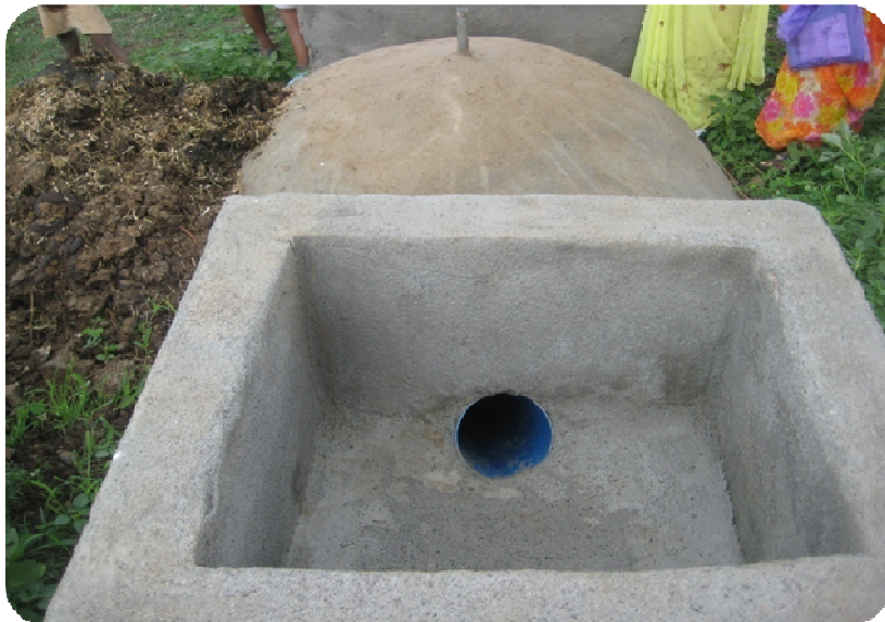
Bio-gas plant, block Bamaniya
